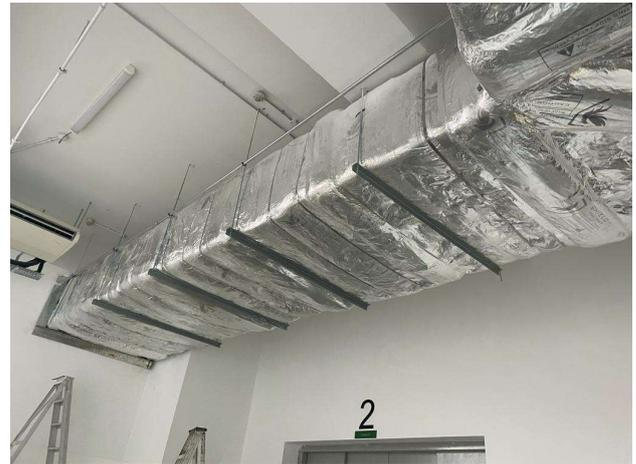
Figure 1: Fire wrap on ducting
