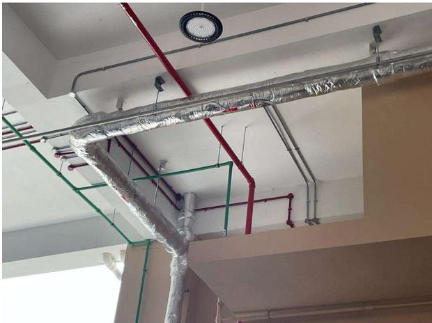
Figure 1: Fire wrap on pipes
