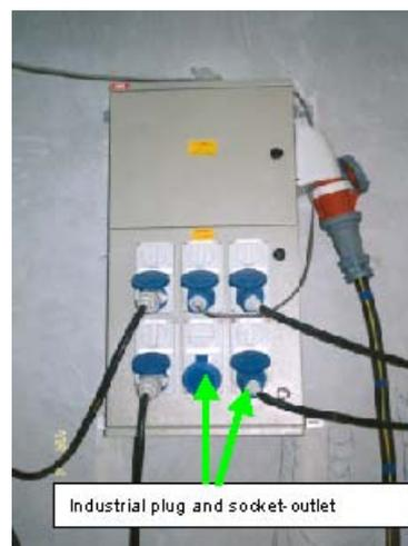
*Fig. 1 – This photograph shows a wall mounted SOA with uncluttered electrical cables connected to industrial socket-outlets using industrial plugs. All live parts are fully enclosed.*
